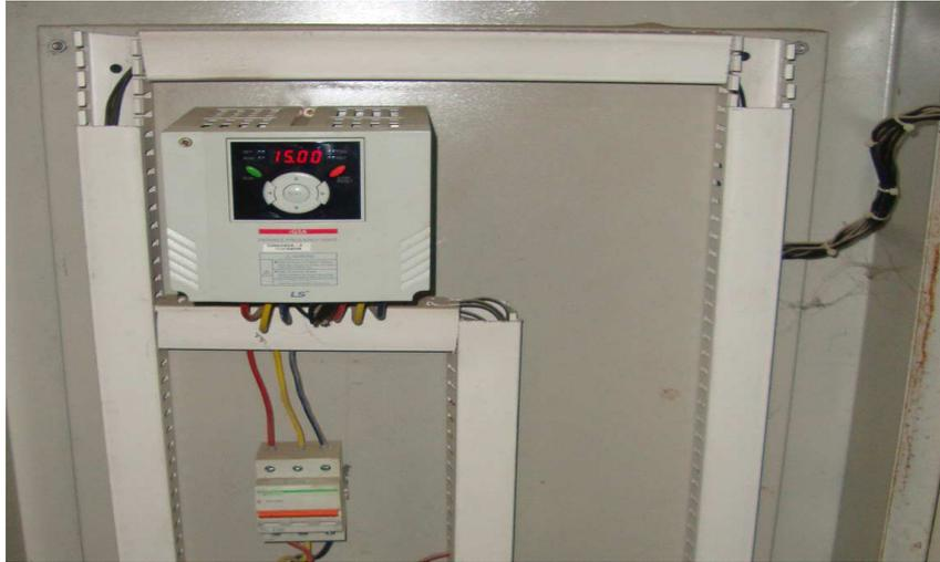
**Photo (5) Wave generator control unit (Inverter circuit)**
